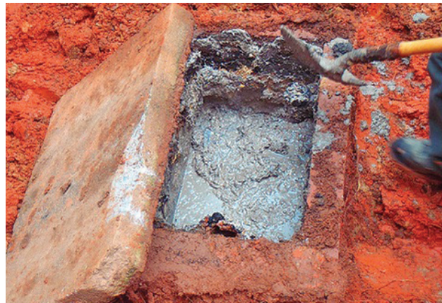
Corroded concrete grease interceptor
