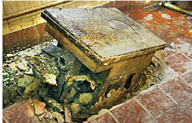
Rusted steel grease interceptor
